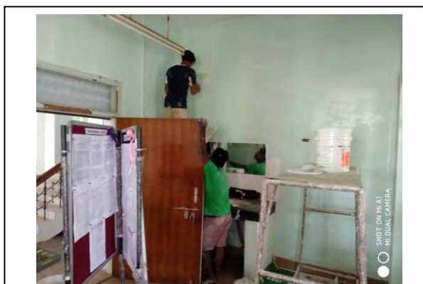
White washing works
