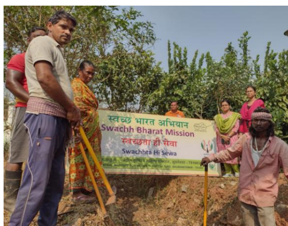
Cleaning of drains in the residential campus
