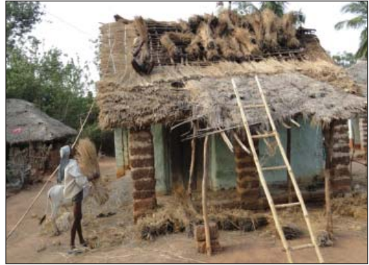
Men undertaking repairing of village hut
