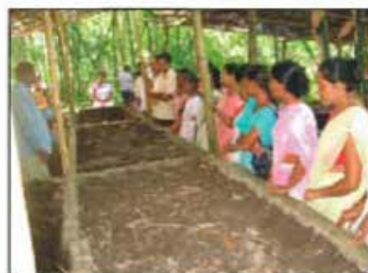
A view of vermi-compost pit under construction
